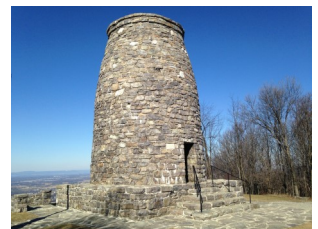
The Washington Monument, atop South Mountain in Boonsboro.
