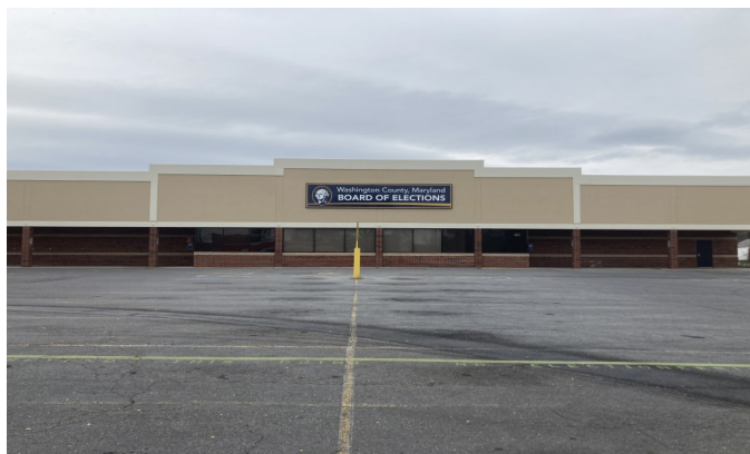
New paint job and sign on front of new facility—11/22/20
