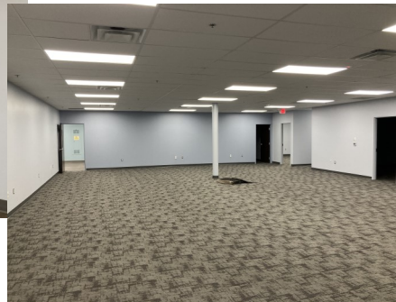
New flooring, ceiling and paint job in office common area.
