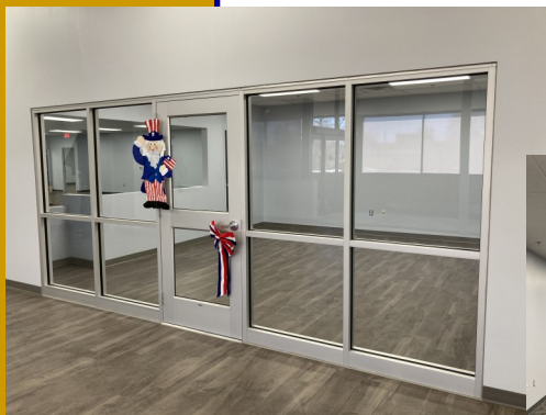
New flooring installed in office lobby area.
