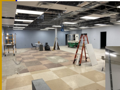
Lighting installed and walls painted in office area—02/01/21
